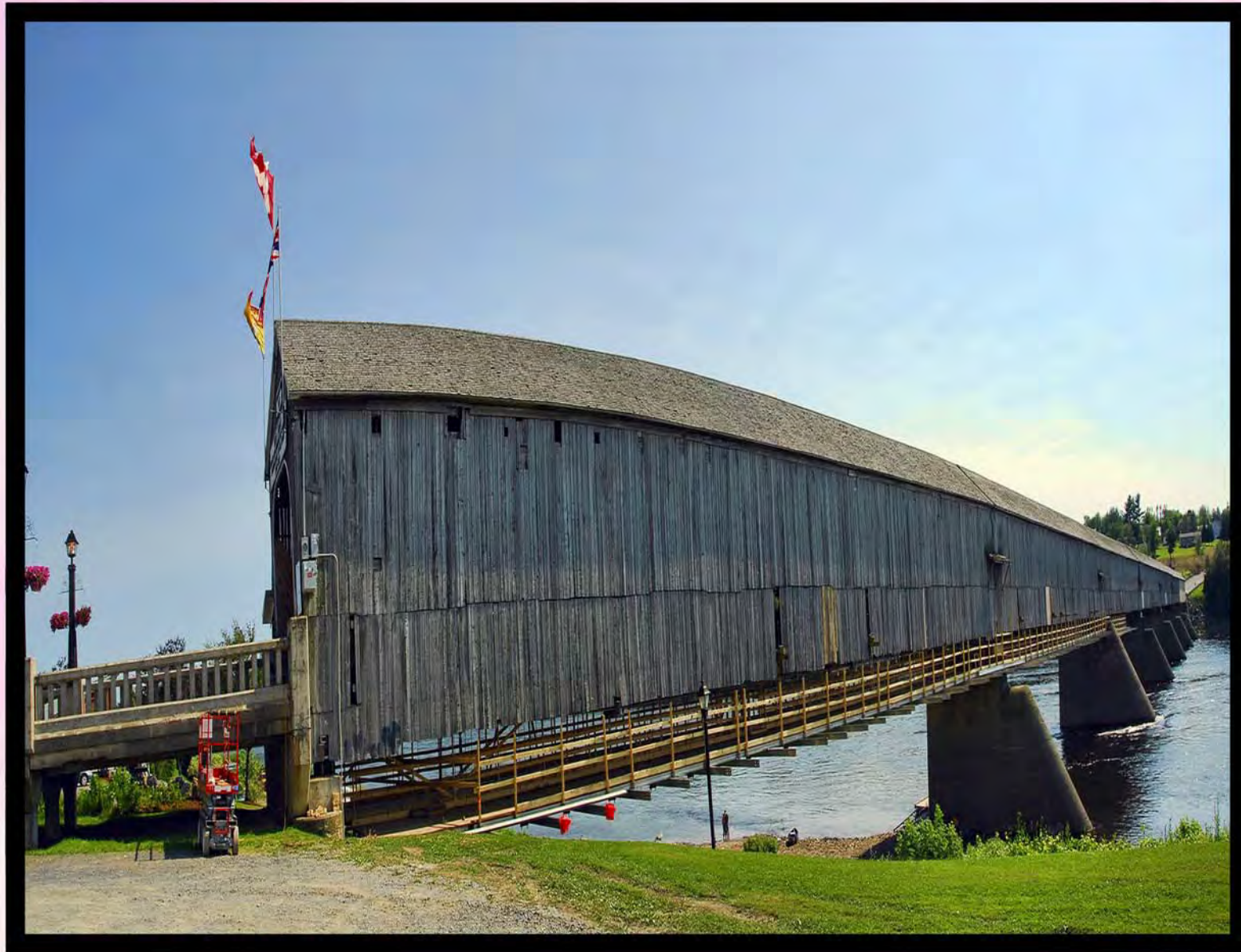
Hartland: New Brunswick Hartland Bridge
