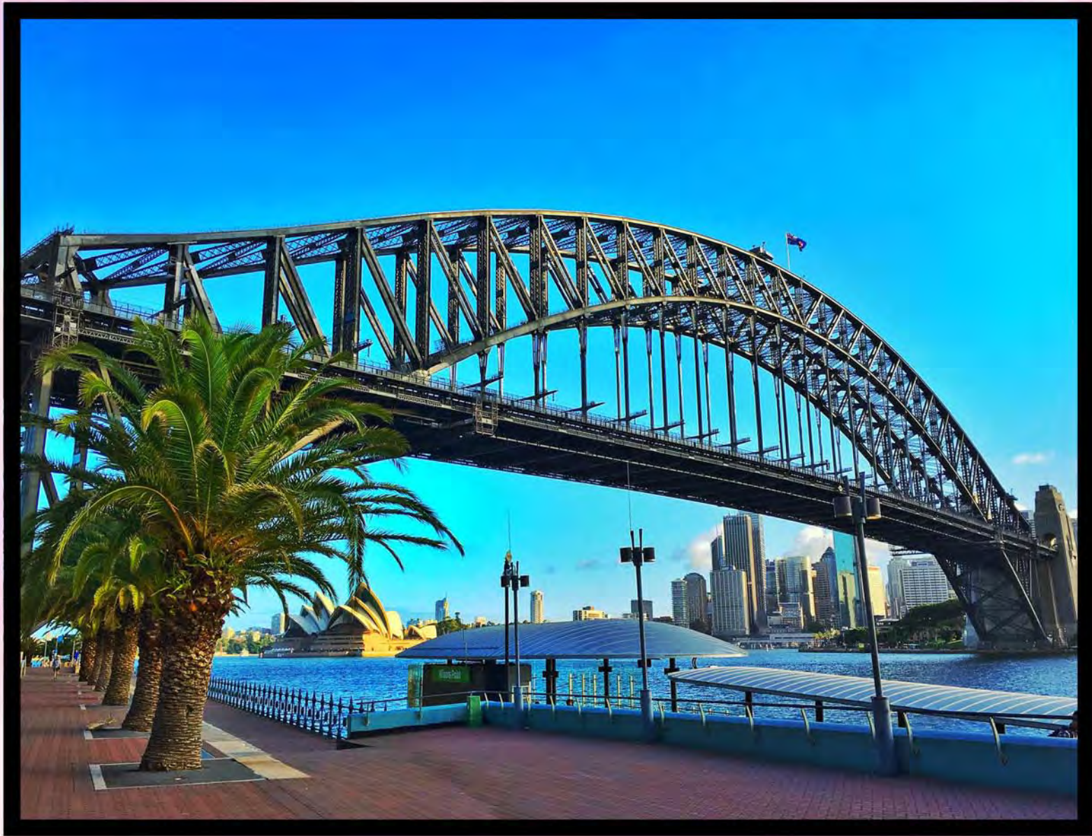
Australia: Sydney Harbour Bridge
